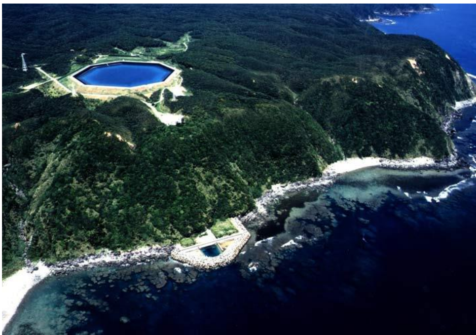
Slika 2.18. Prva RHE koja je koristila morsku vodu u Kunigami, Okinawa, Japan. ( http://blogs.worldwatch.org/revolt/pump-up-that-seawater-a-remix-to-pumped-storage-hydro/ pristupio 10.5.2017)
