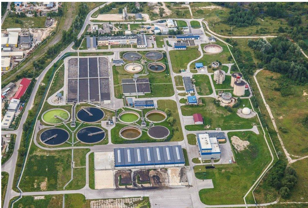
Figure 7. Wastewater treatment plant viewed from above, showing typical bioreactors (rectangles) and sedimentation tanks (circles) [73]
