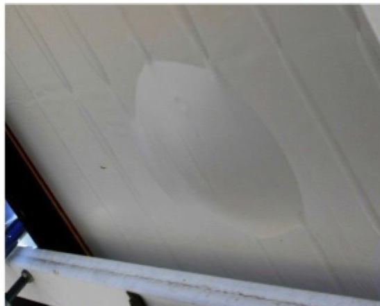
Figure 2.7. Delamination of backsheet [11]
